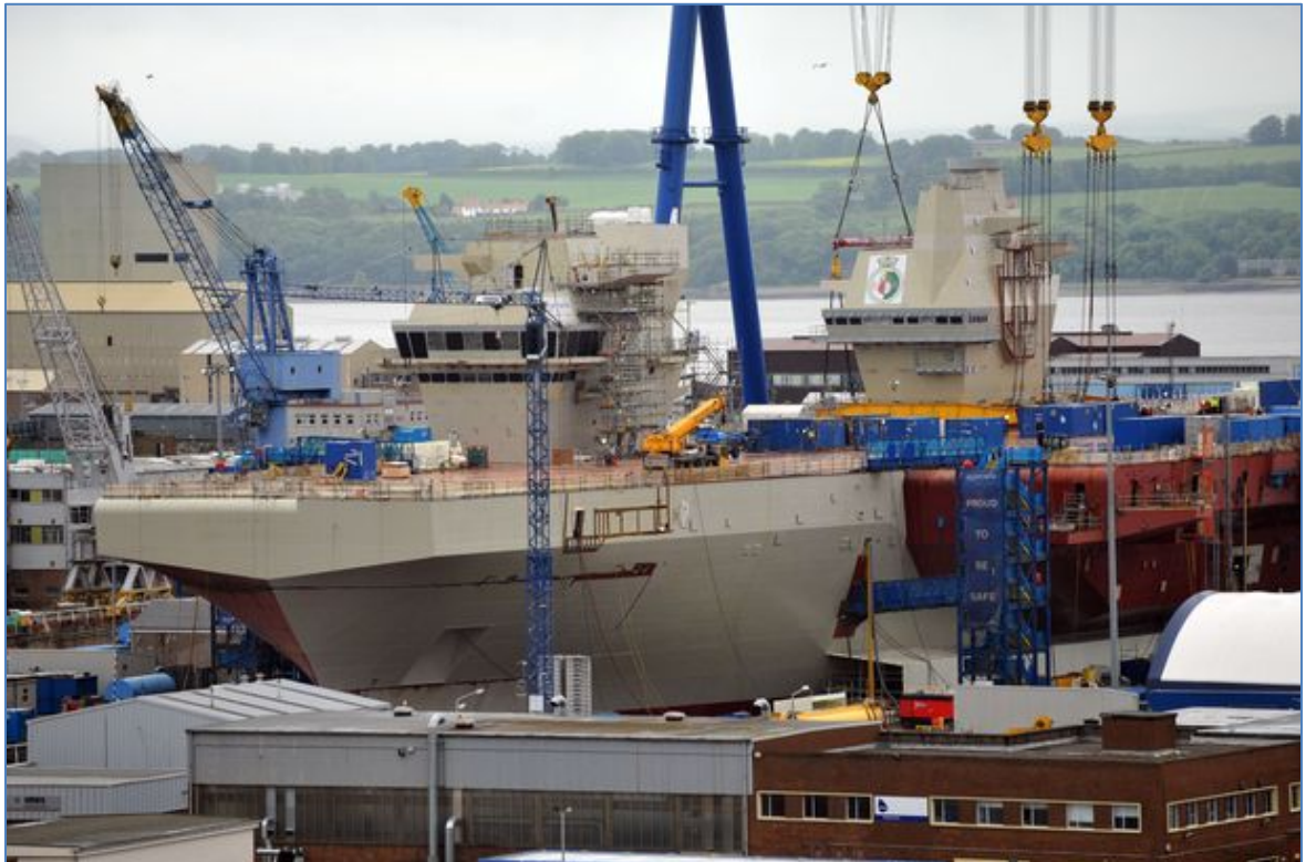
Figure 2 – HMS Queen Elizabeth under construction (photograph by Phil Dye).
